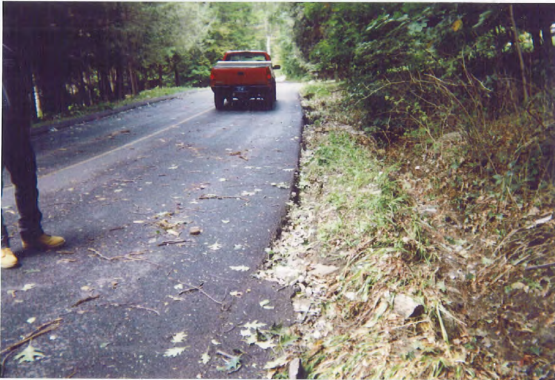
Rocky Hill Road. Eroded and undermined at the edge of the pavement. Typical of several areas at this road.
