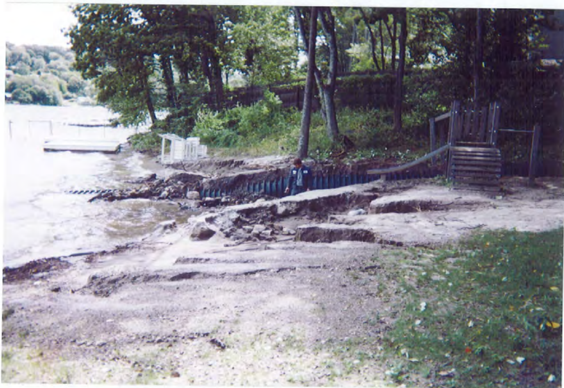
South Beach area showing major erosion of sand and earth. Pipe has been exposed and lifted out of the trench.
