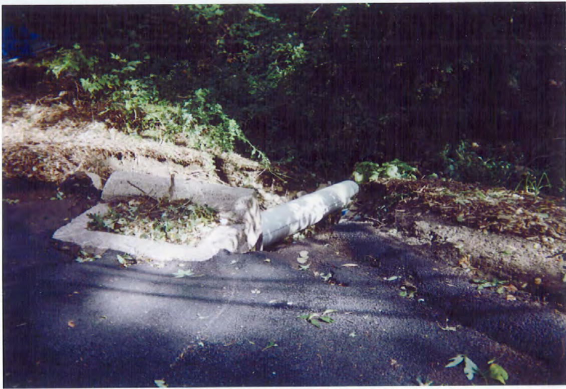
Bigelow Road: shoulder, pavement washed out, pipe exposed. This is typical of many areas.
