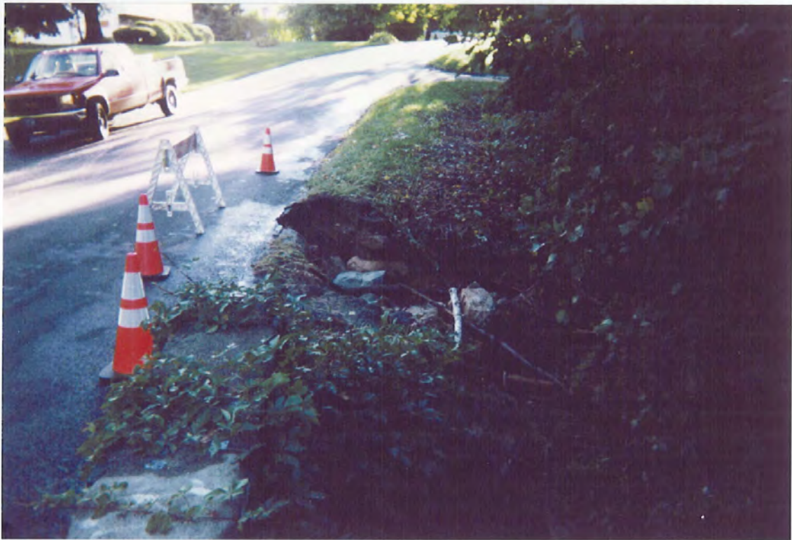
Old Farm Road at the culvert. The headwall has washed away.
