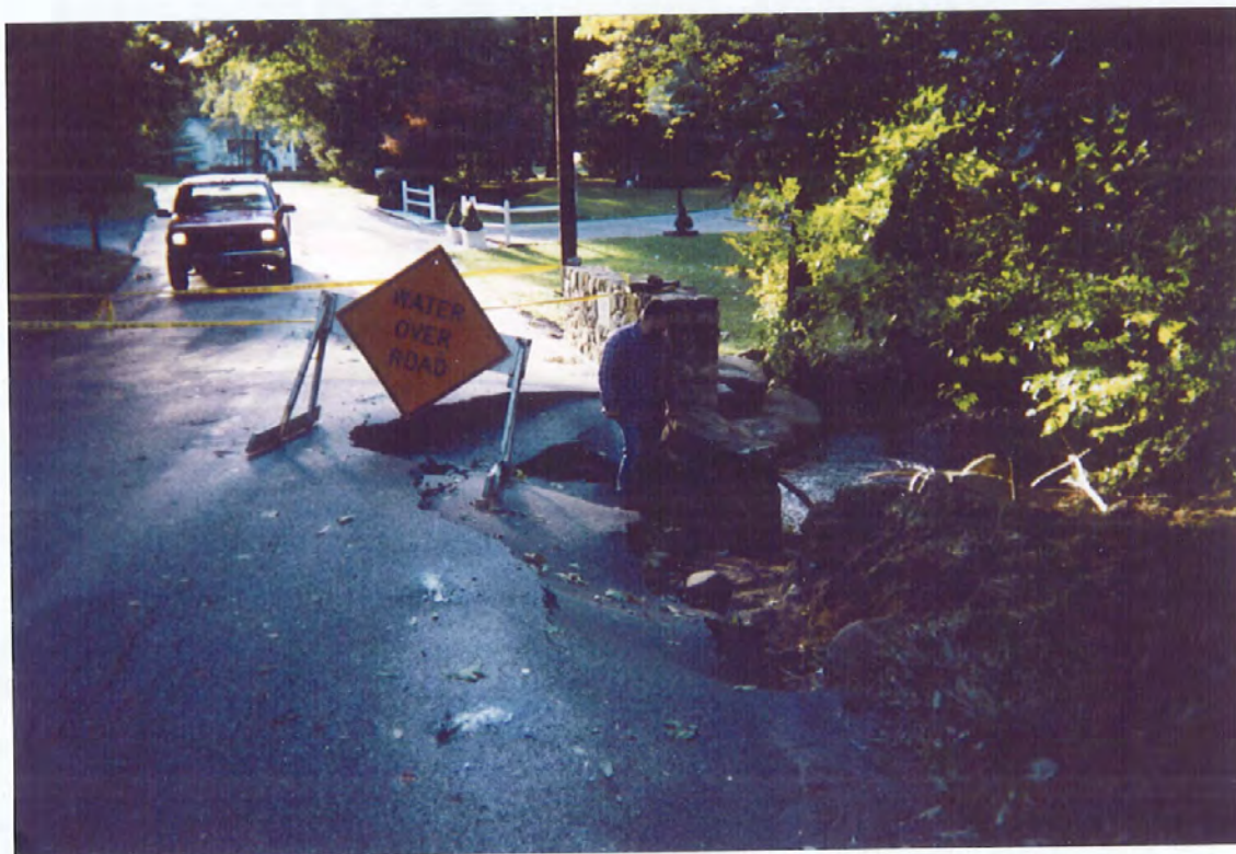
Second view of Smoke Hill. The headwall is gone. Drainage is exposed.
