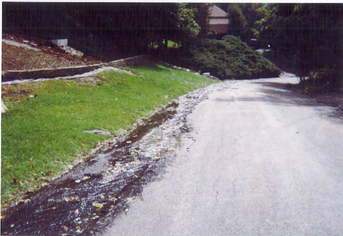
Woods Way, where the water caused up to four layers of asphalt to rip apart.
