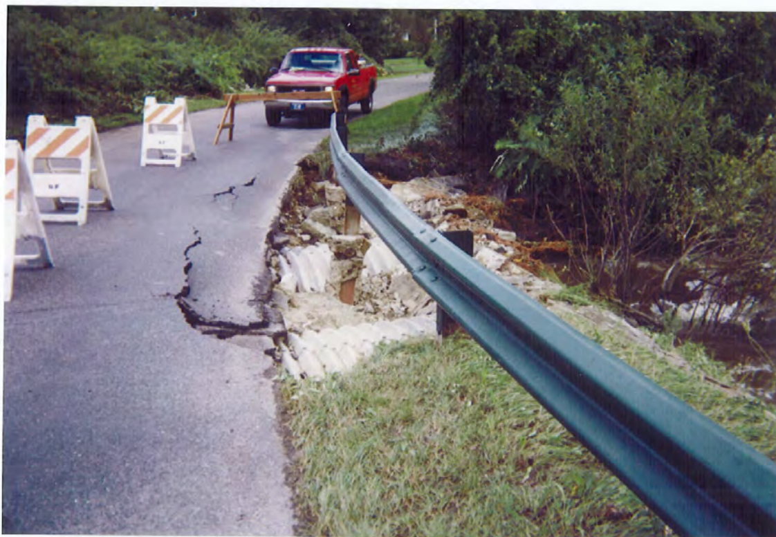
Musket Ridge Road. Three 60 inch pipes could not handle the water. The headwall at the outlet is gone, the shoulder and one lane of the road is heavily damaged.
