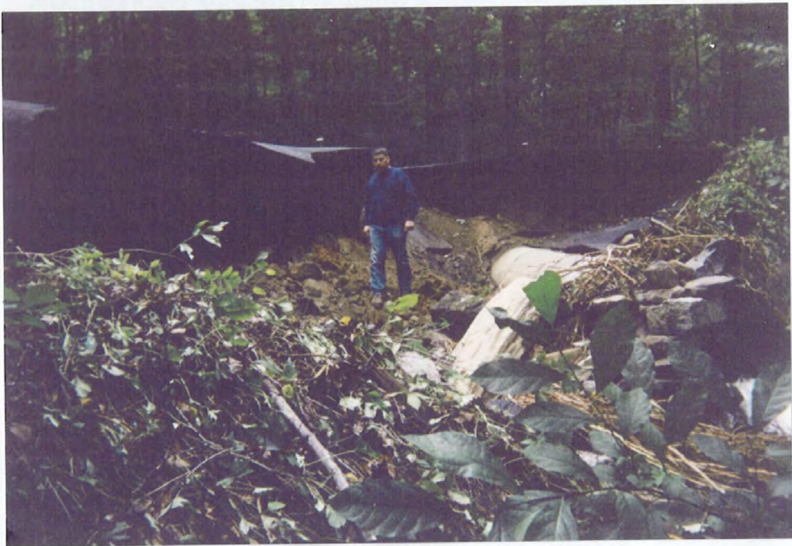
Beaver Bog Area 1. Where I am standing the pavement should be one foot over my head
