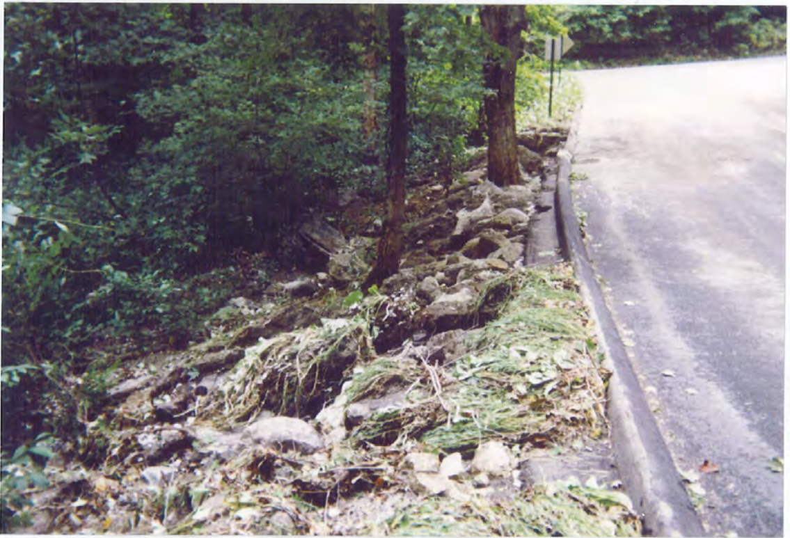
Area of Rocky Hill Road where the water flowed over the road, destroying the shoulder. If rains continued this would be collapsed similar to Beaver Bog.
