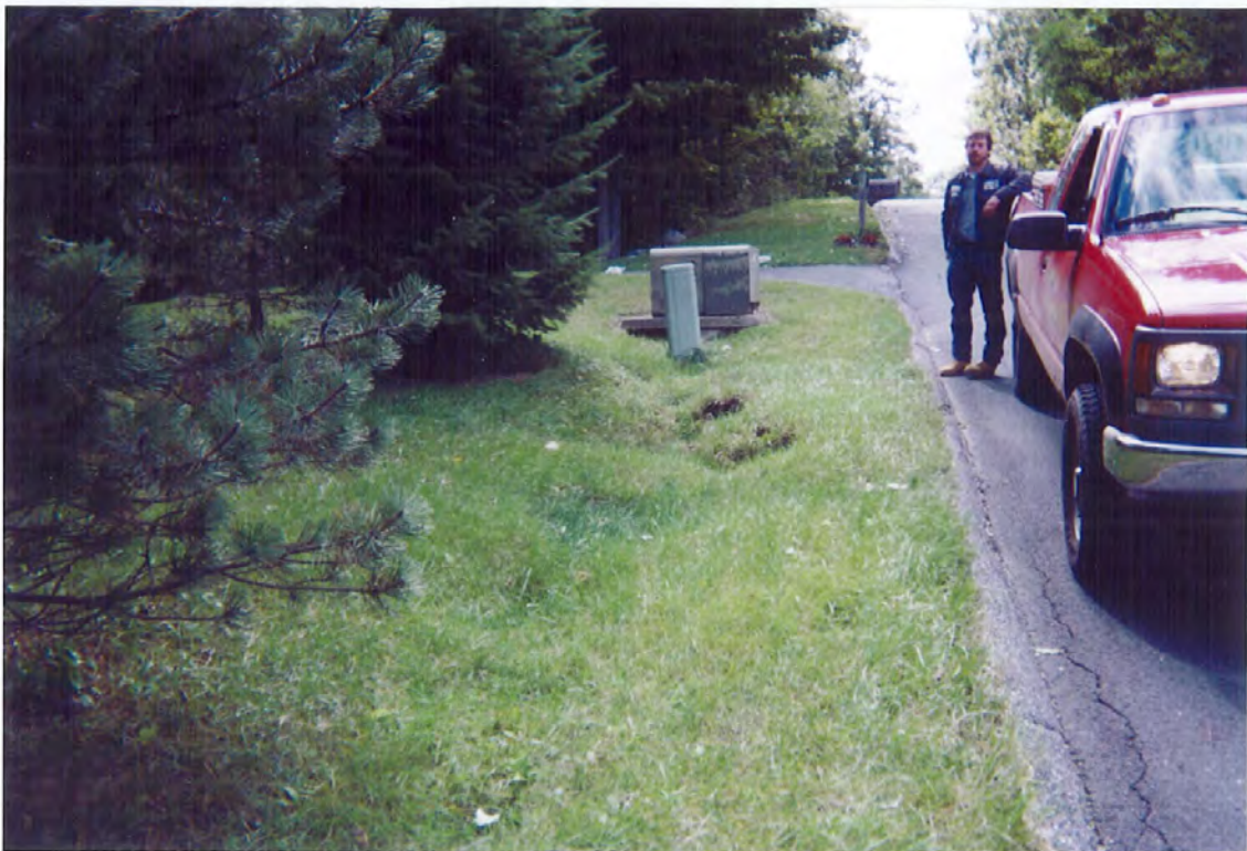
Jennifer Drive. Water was so severe that utility trench acted as a curtain drain, causing sink holes directly over utilities.
