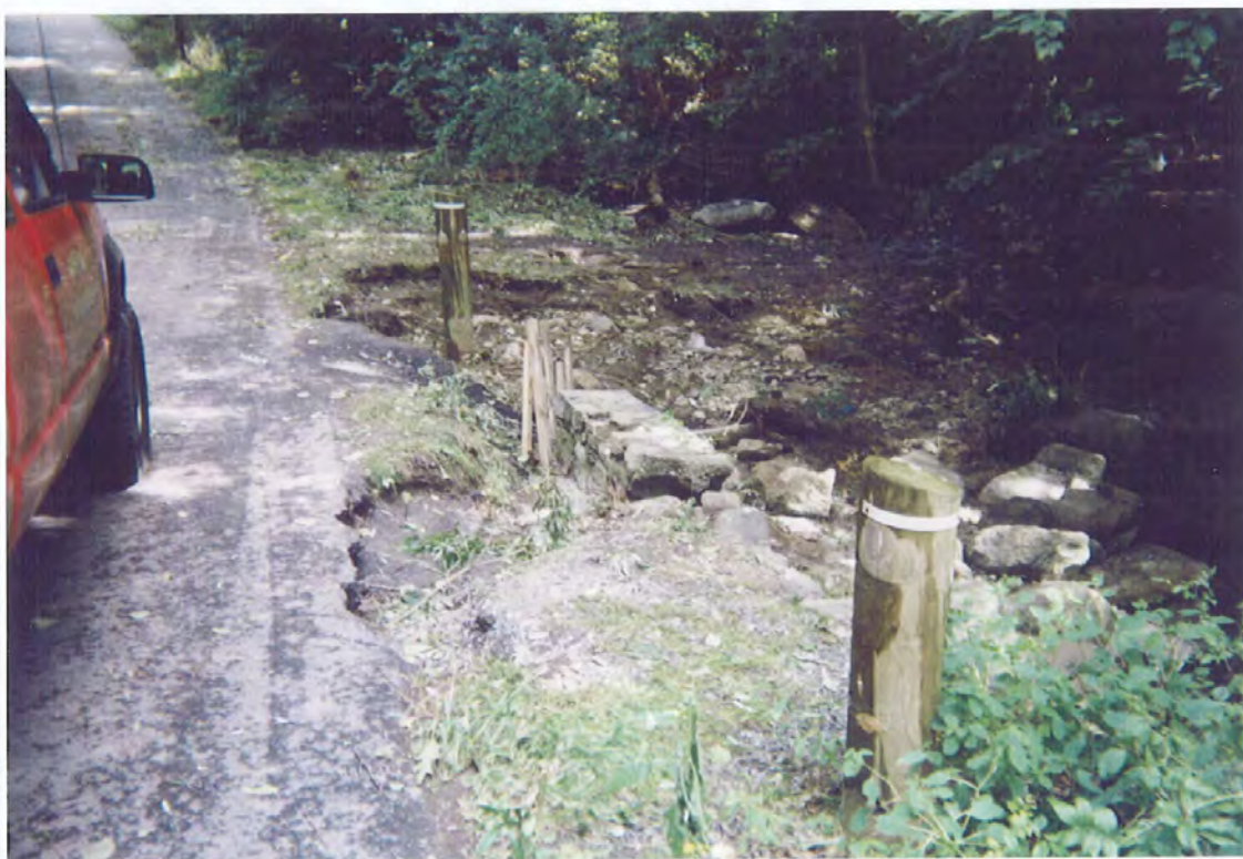
Brookside Drive where the culvert has washed out. Shoulder, pavement and headwall damaged.
