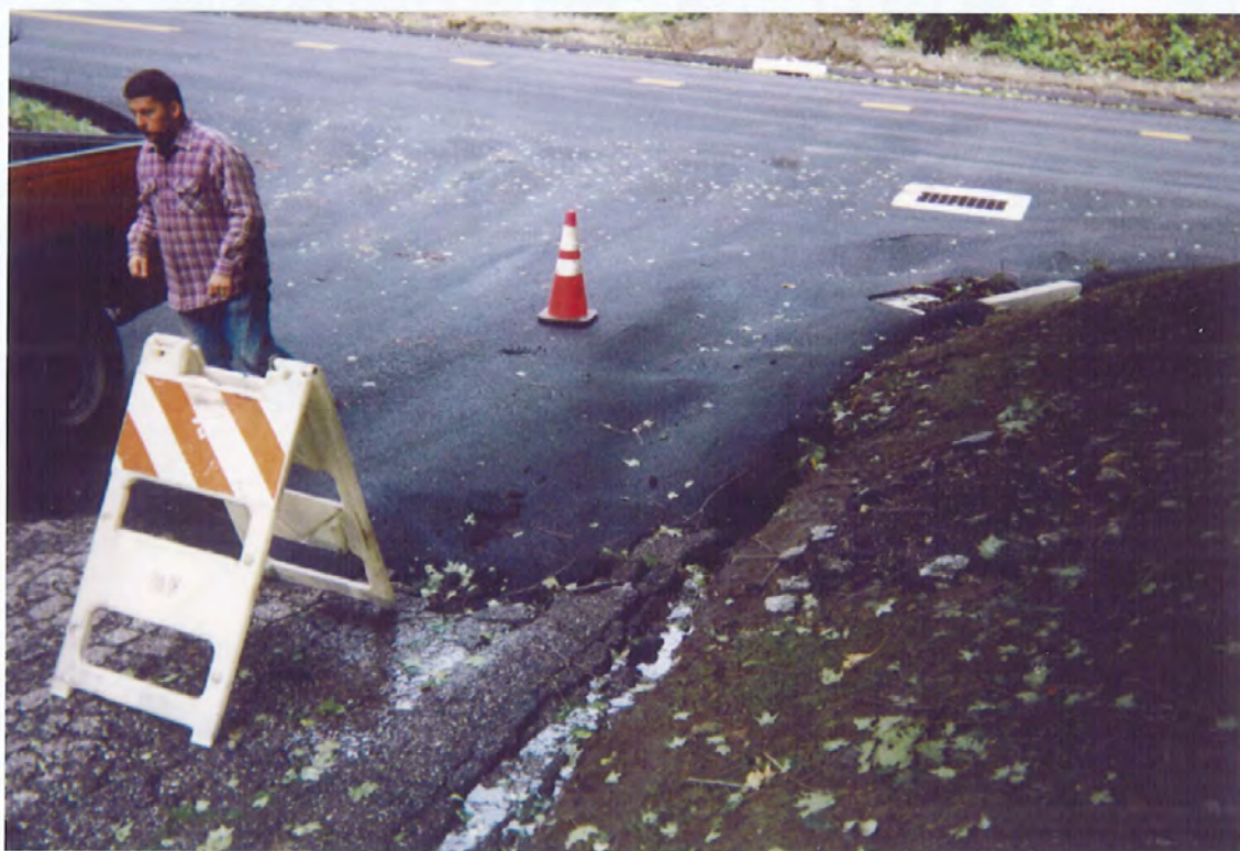
Intersection of Meeting House Circle, where the pavement is buckled and undermined. Note how the silt has pushed the pavement up around the catch basin.
