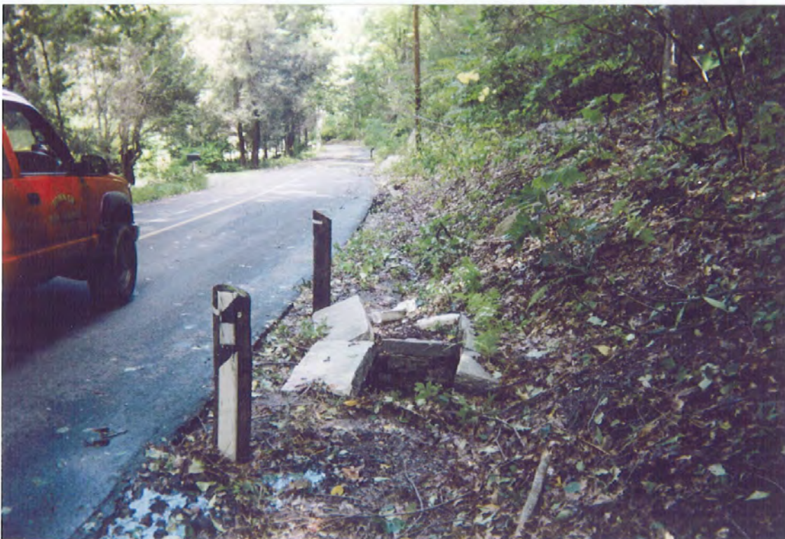
Catch basin on Shortwoods Road which has been collapsed due to water.
