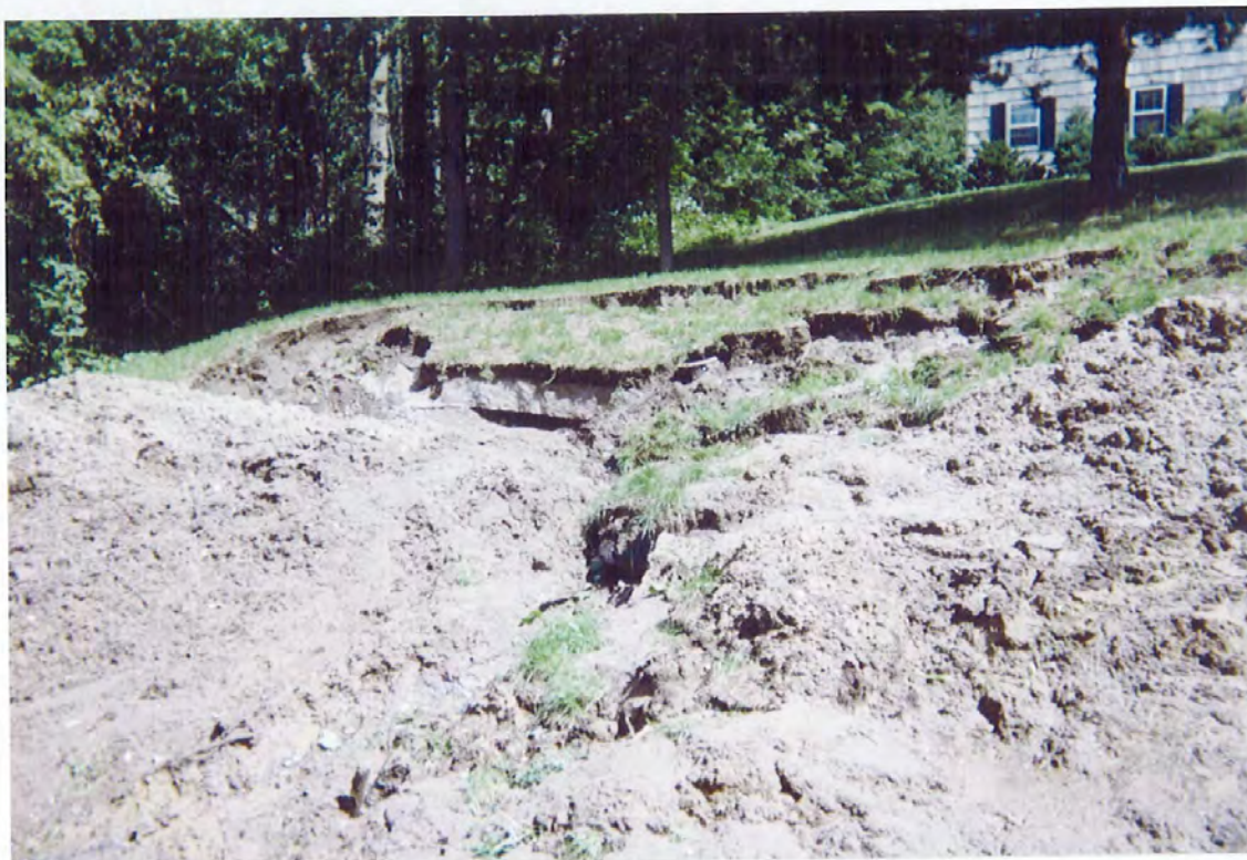
Complete septic failure and washout at Paradise Court. This photo was taken after the Highway Department removed two feet of topsoil, silt and septic sand from the road.
