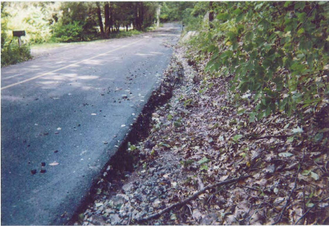
One of several areas on Shortwoods Road that are washed out. Pavement is undermined 18 inches into the travel lane. This is the typical type of damage at approximately 30 other locations
