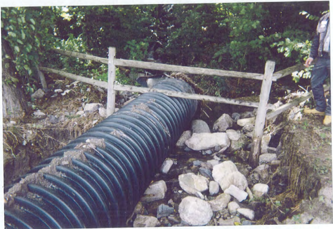
Third view of South Beach. The pipe has floated high enough to dislodge the fence.
