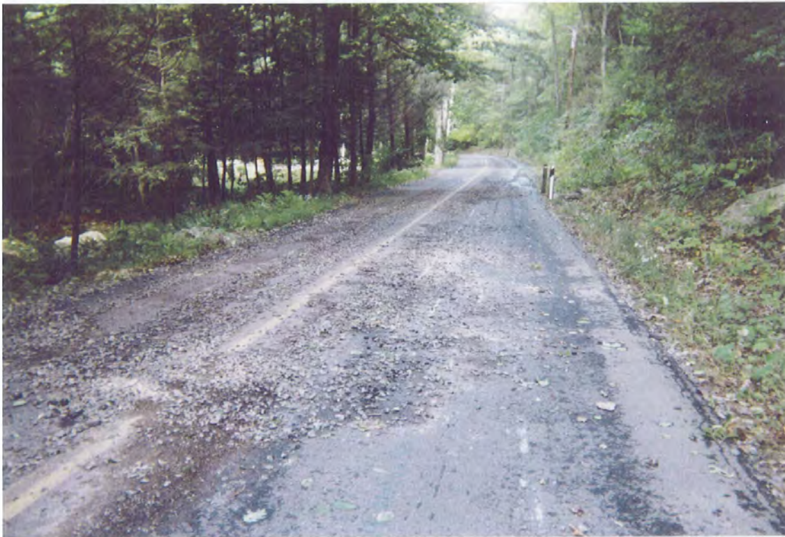
Area of Shortwoods Road where all the stone from a curtain drain has been washed out of its trench. Approximately 100 cubic yards could not be removed.
