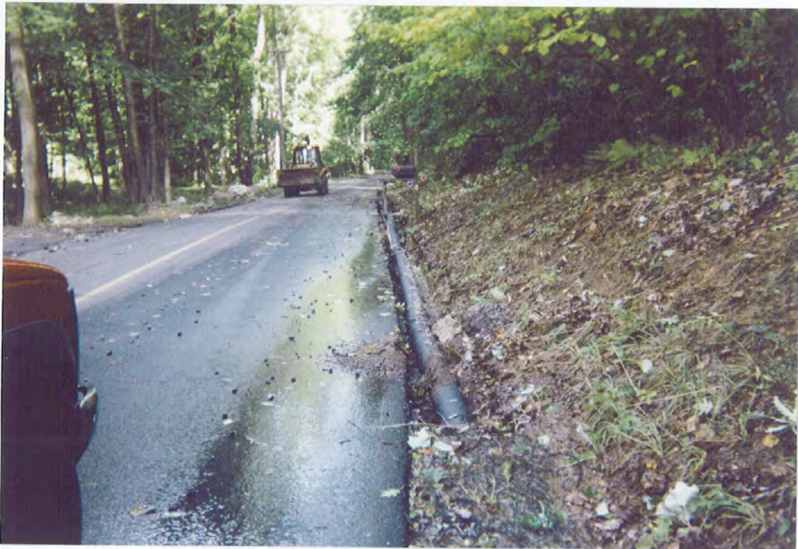
Second view of exposed curtain drain on Shortwoods Road.
