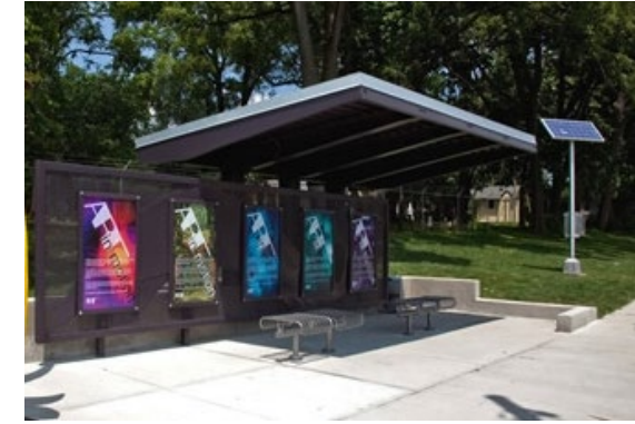
Bus stops in Lexington, Kentucky, using solar technology for lighting enhancing public safety as well as public health
