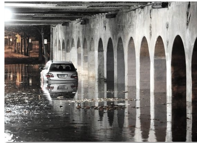
Superstorm Sandy, Humphrey St. Underpass
